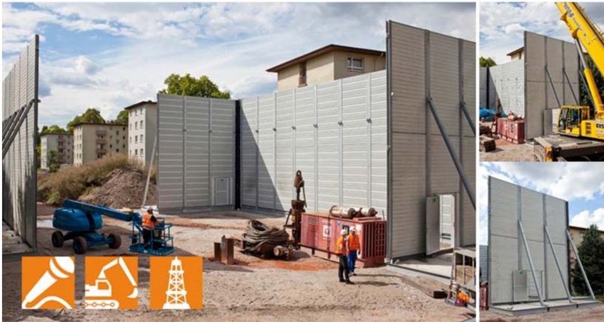
Figure 11.5: Temporary Screens for Use during Construction
